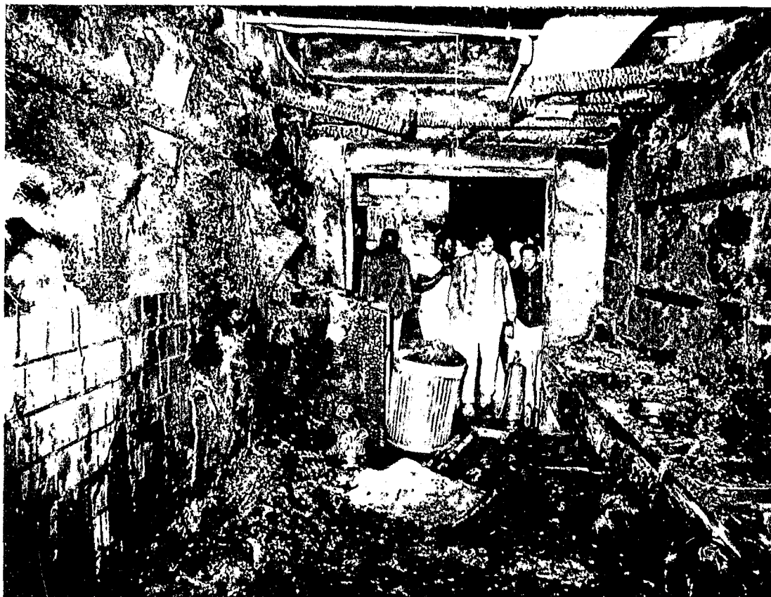
This washroom in the Danbury, Connecticut correctional facility was near the primary means of egress from the dormitory. The fire's initial growth, with flame spread and heavy smoke, was due to fiberglass reinforced plastic wall paneling and its plywood backing. (Credit: John Mongillo, Jr., New Haven Register)
