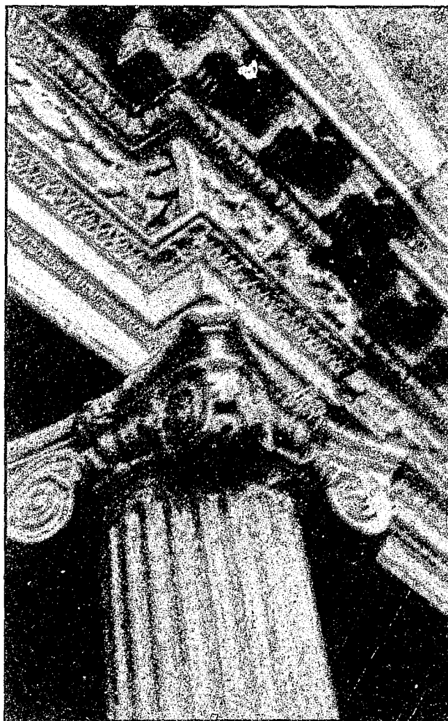
Column in the Statehouse, Annapolis
