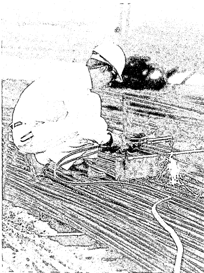
Reinforcement bars being cut at a construction site.
