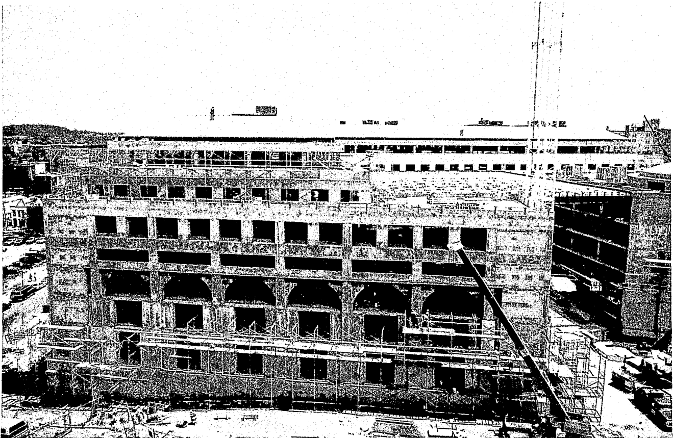
The pace of construction on the Judiciary Office Building has been brisk; the building is shown here in July 1991. The photographer's vantage point is the parking garage of Union Station.
