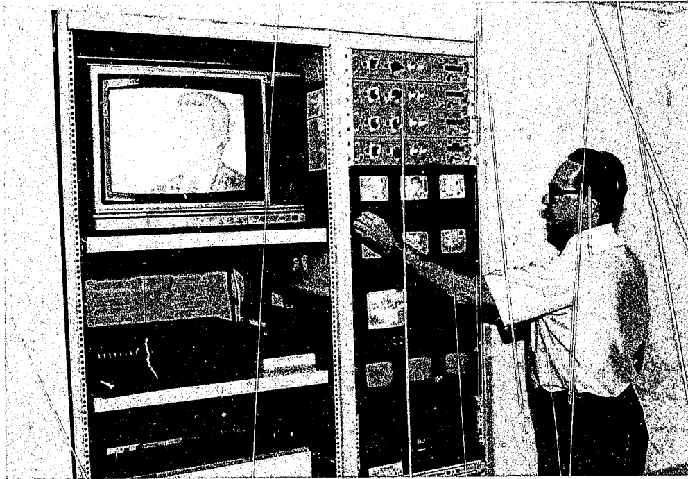
FIGURE 6-2. TELEVISION MONITORS AND VIDEO RECORDERS IN OPERATIONS AREA
