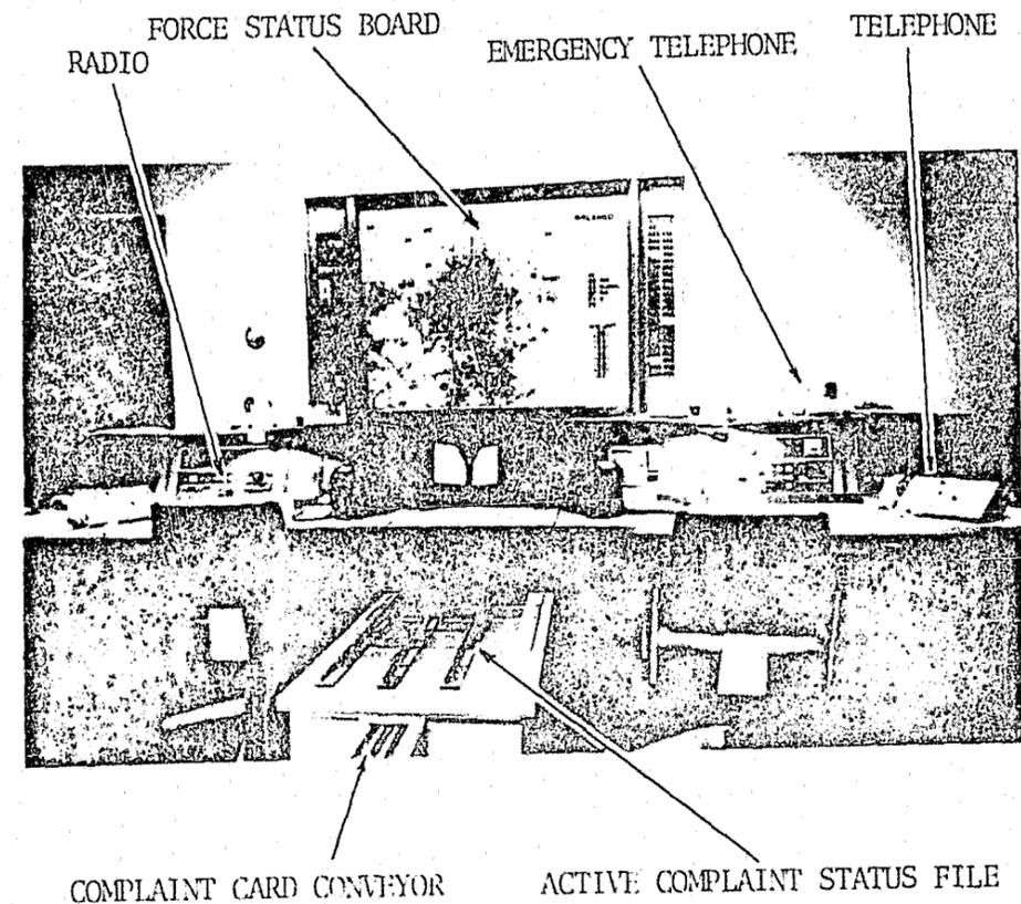
Figure 10 Photograph Of The Radio Operator Work Station Showing Major Equipment Position.
