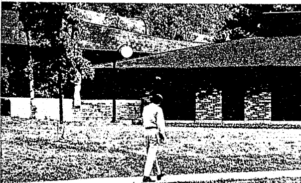
A model institution now in operation. The campus like Robert F. Kennedy Youth Center in Morgantown, West Virginia, a minimum custody facility, is the federal government's first especially designed to facilitate treatment of a youthful population. Its program puts the accent on the individual; the 300 16- to 20-year old "students" may start at their own levels of learning and go as far as they wish. Only one of the four housing units—or cottages—has built-in security features. In such an open institution, escapes are expected; however, each is studied in order to find the underlying causes and to develop methods by which to reduce them. The center serves, as will other federal institutions now being planned, as a research and learning laboratory and as a model for other correctional systems. Architects: C. E. Sillling & Associates; associate architects: Schmidt, Garden & Erickson.
