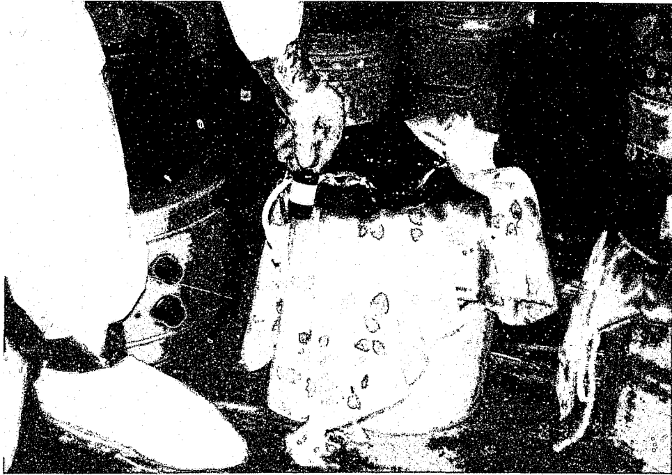
Gravity filter setup. Note bedsheet used as filter.
