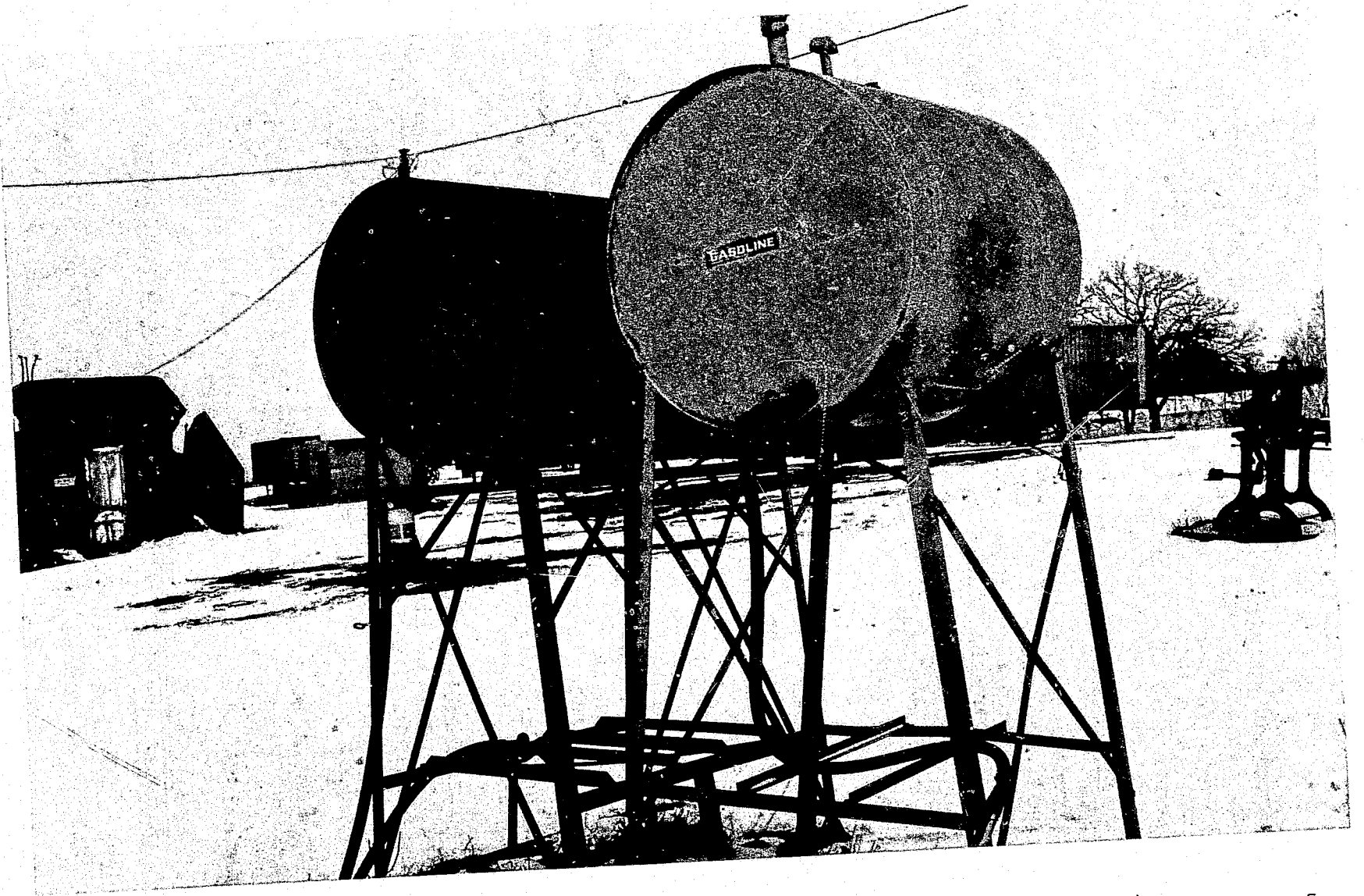
Gravity feed gasoline tanks without proper shut-off valves, on the premises of the inoperative New Melrose Fireworks Display Company plant. Photograph courtesy of the Illinois State Fire Marshal's Office.
