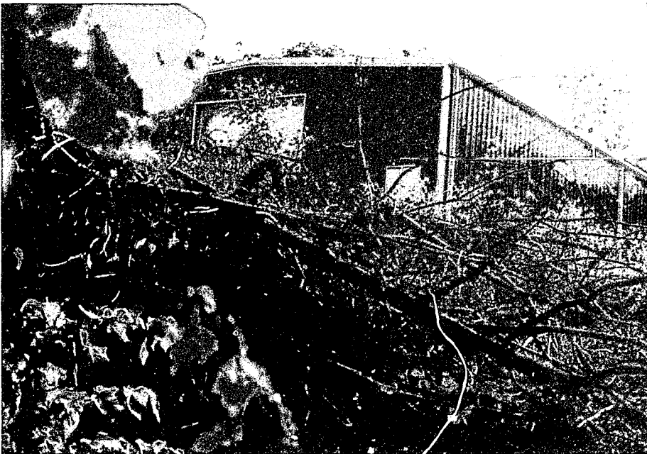
40' x 80' metal building as seen from woodpile which concealed exhaust heat and air intake.
