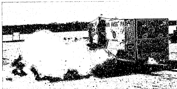
An explosive test on a baggage compartment.
