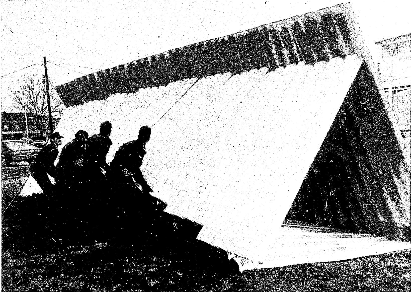
Figure 13. Feasibility Test of the Corrugated Aluminum Panel Riot Barrier Showing the Initial Phase in Turning over the Barrier.
