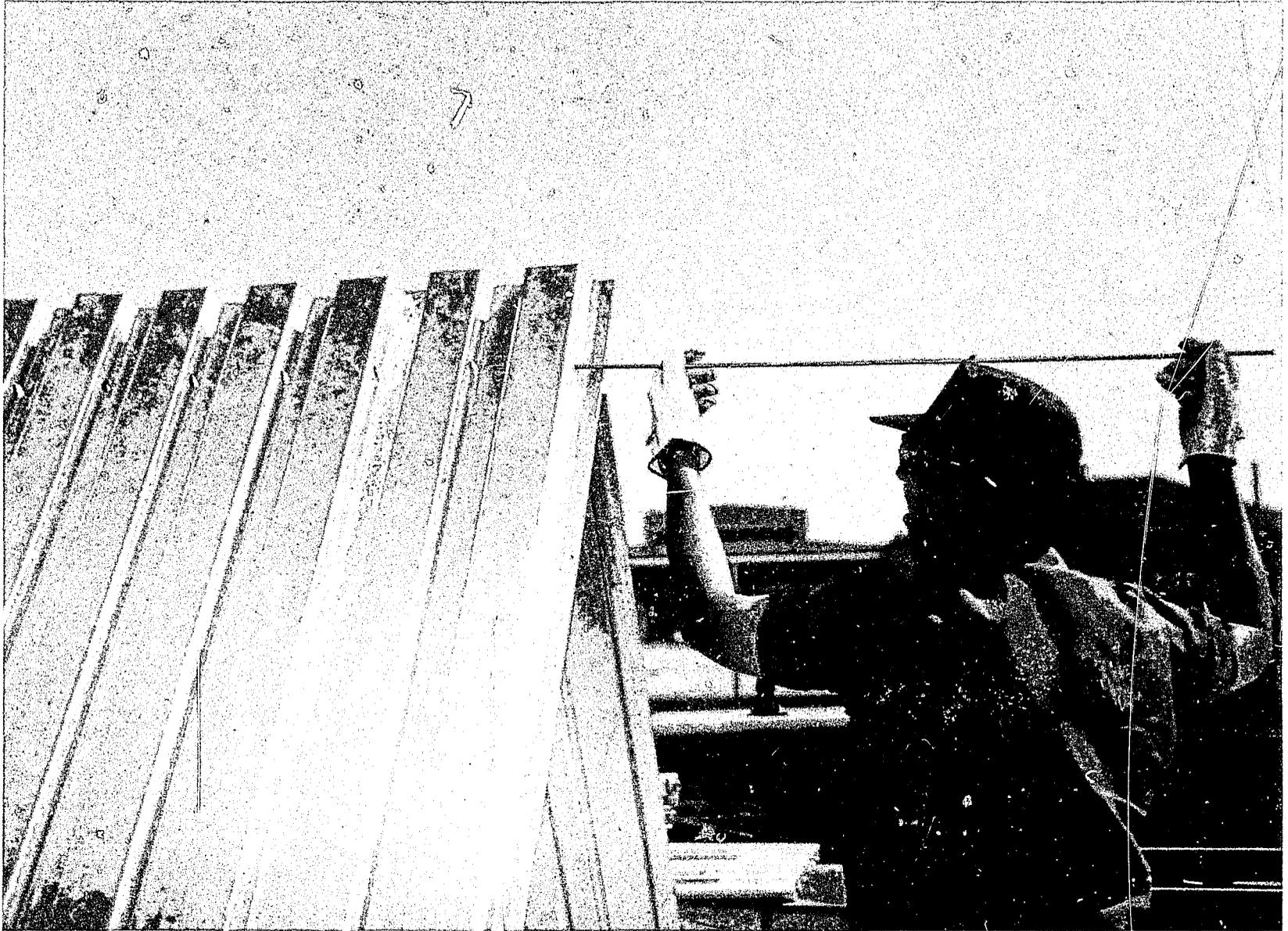
Figure 3. Pin Connection of the Apex of the Two Sides
