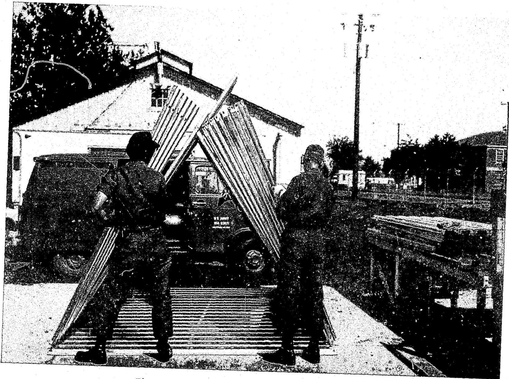
Figure 2. A Collapsible Module being Erected.
