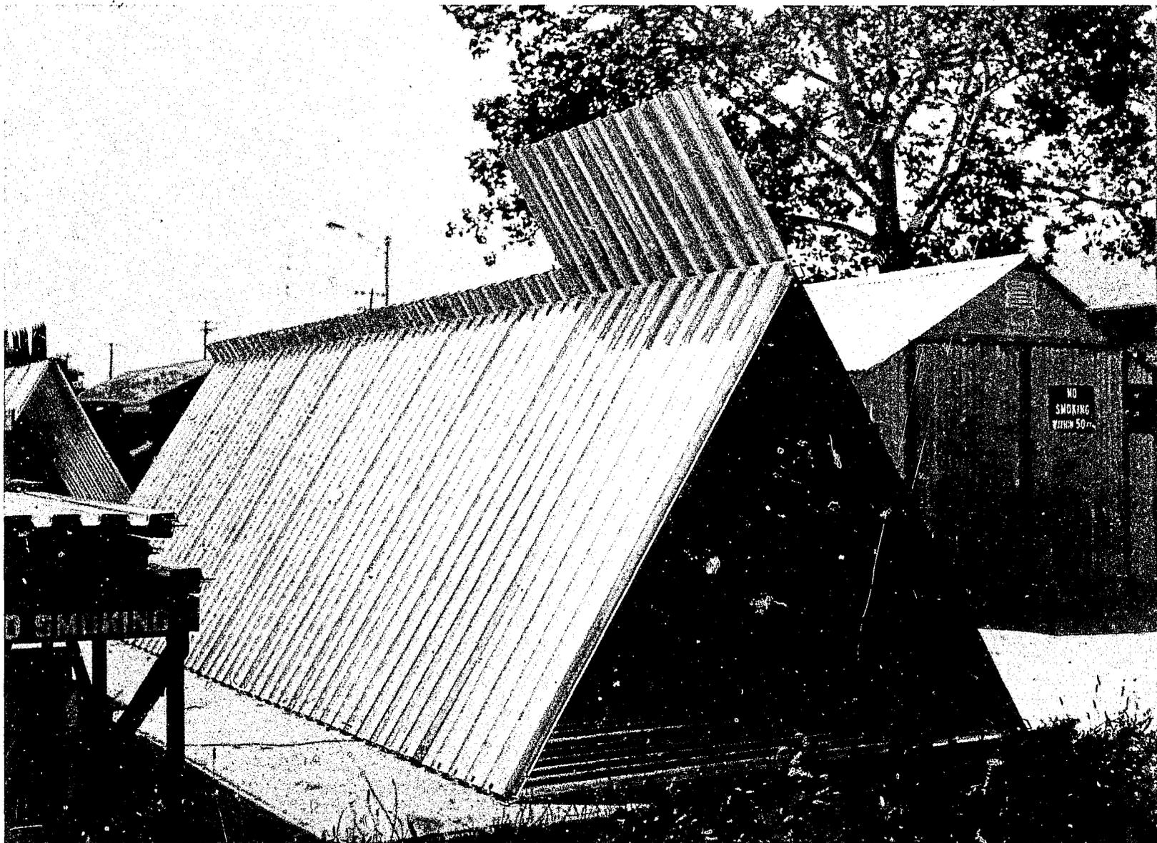
Figure 4. Comparison of Modules With and Without the 2-foot Extension to One Side.
