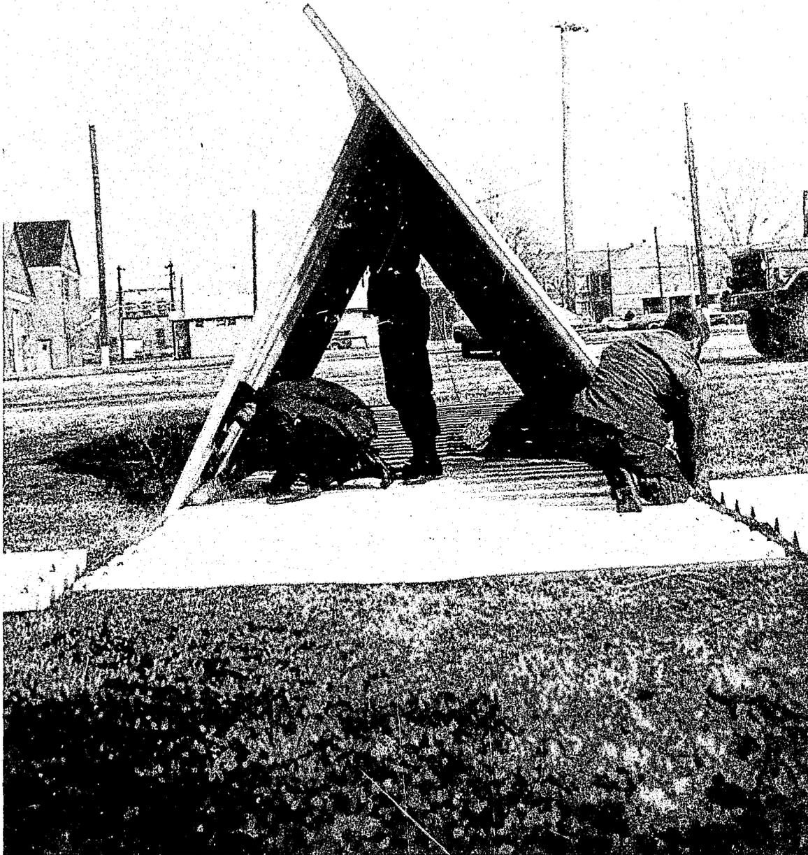
Figure 6. Assembly of Corrugated Aluminum Panels Using Wire Cables for Fastening.
