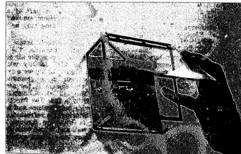
FIGURE 11. Plastic box to protect master control switch against inadvertent operation. Photograph courtesy of Shell Oil Company
