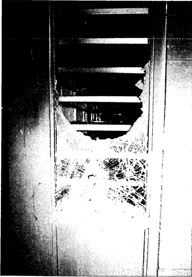
Figure 9-2 The Control center in ISCI's Unit 9, into which this window looks, was destroyed by inmates during the 1988 riot. While the bars on the windows were not broken, inmates were able to gain access to the Control Center by breaking holes in the cinderblock walls. Source: Department of Correction, State of Idaho.
