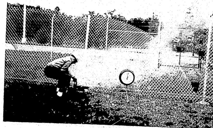
Figure 170. Abrasive Wheel Saw Used to Cut Nearly Full Height of Fabric and also to Cut Off One Intermediate Post; Test F1
