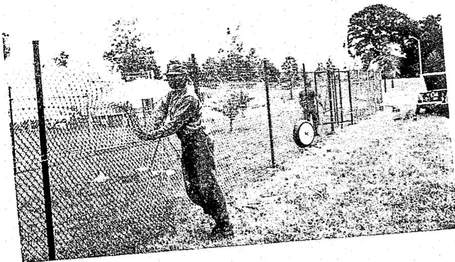
Figure 184. Pulling Down Fabric from
