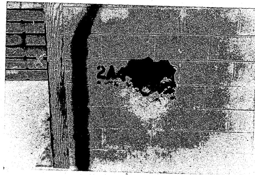
Figure 13. Initial 3" Diameter Breakthrough
