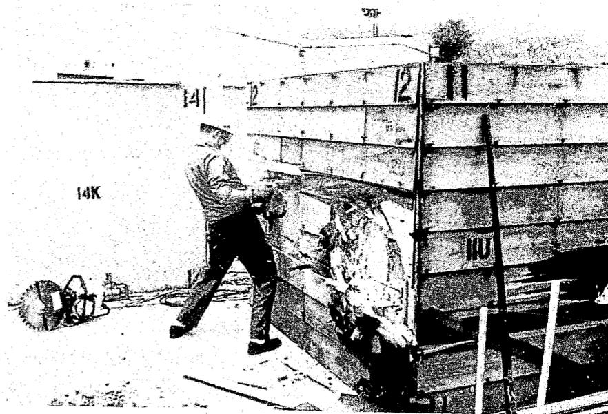
Figure 102. Cutting with Hubless Saw; Test 12
