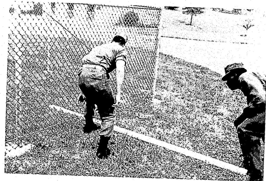
Figure 173. Placing 2 X 4 in Position;
