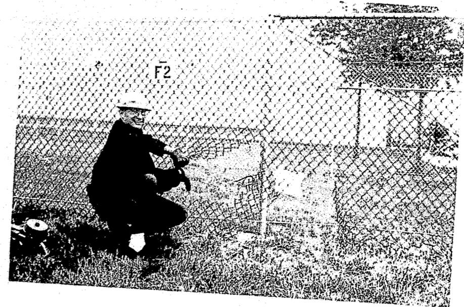
Figure 179. Opening Produced by Abrasive Wheel Saw; Test F2
