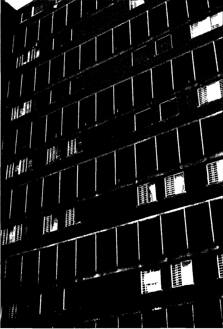
Photo 5. Lake Street Building, Henry Horner Homes. Photo by Jean Amendolia.
