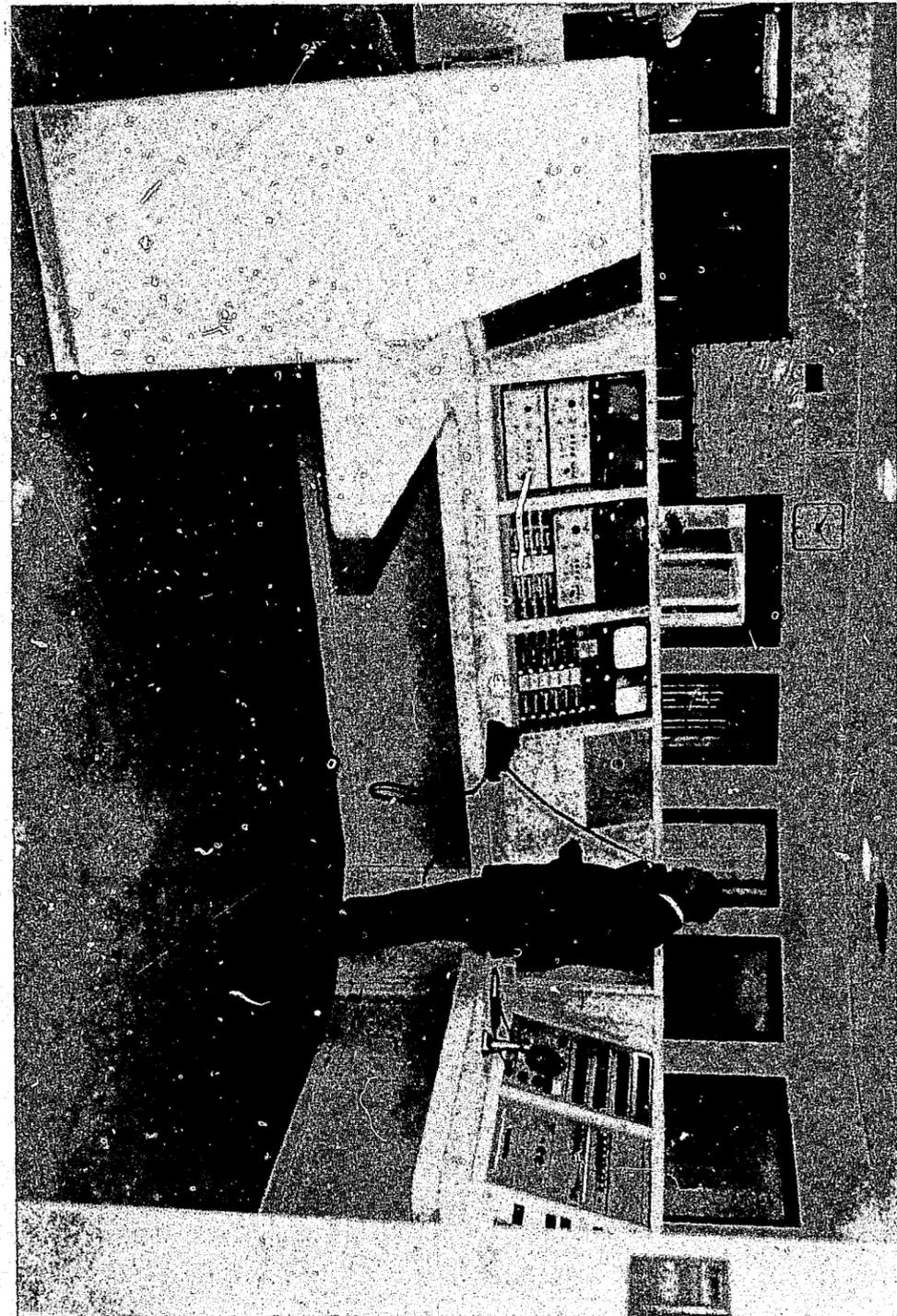
Sheriff Joseph A. Smith before the closed circuit TV monitors of Central Control which serves as the nerve center of the entire institution. Central Control's main panels also contain a 4-channel AM-FM radio console, supplying music to every cell; a complete radio mobile communications unit; a multi-purpose intercom system; heating, electrical, and air conditioning monitors; and controls for all electrical traps and corridor barriers.
