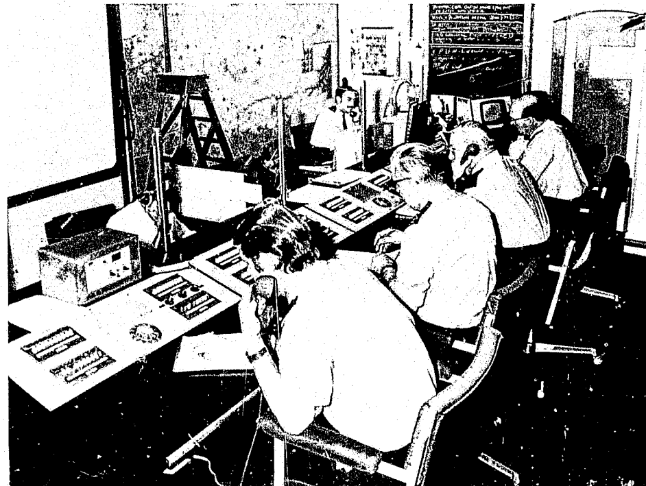
Force Headquarters Control Room.
