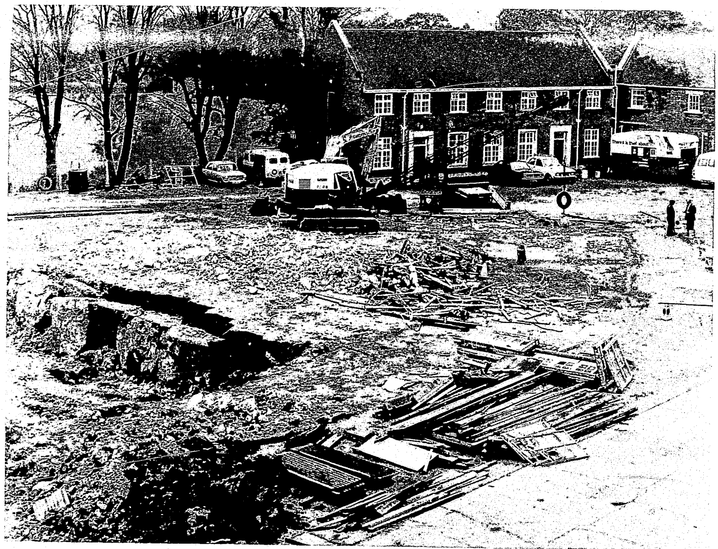
Site clearance at Force Headquarters in preparation for the building of the new Communication, Office and Amenity Block.
