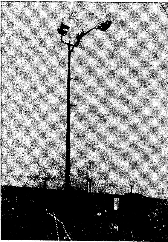
FIG. 3-12 SIGNPOST MOUNTED ON A LIGHTING STANDARD
