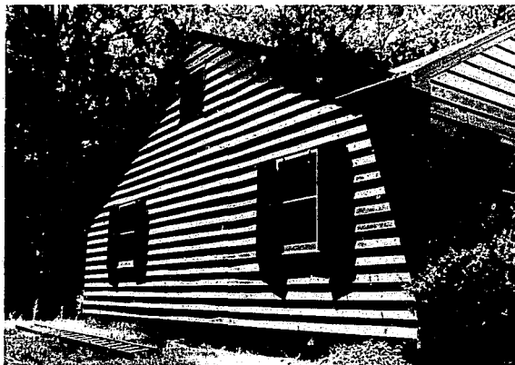
FIGURE B-3. East end of test house. (a) Conventional photograph.
