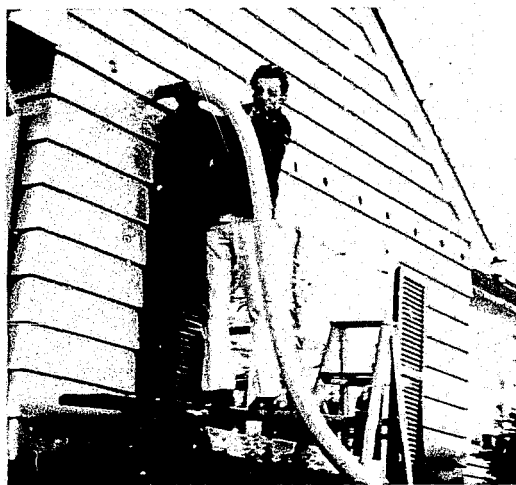
FIGURE A-4. Glass fiber being blown into a wall section.
