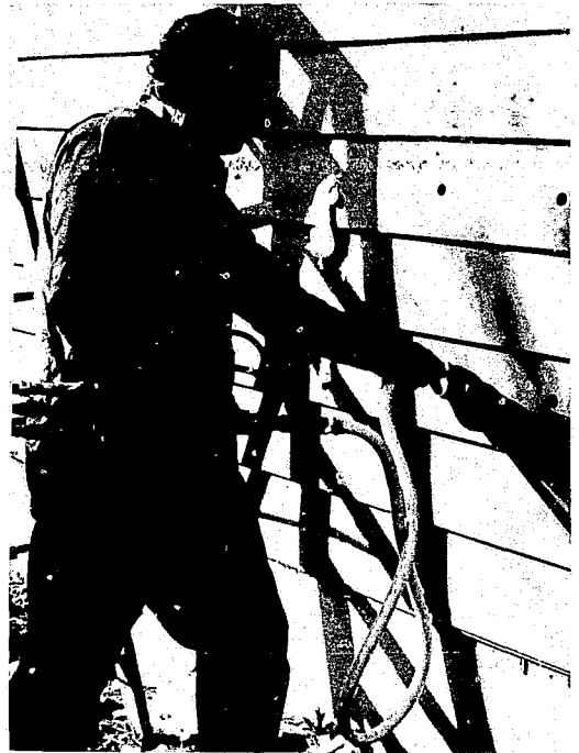
FIGURE A-5. Urea-formaldehyde foam being blown into a wall section.
