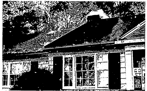
FIGURE C-4. Major air leakage path through the chimney.
