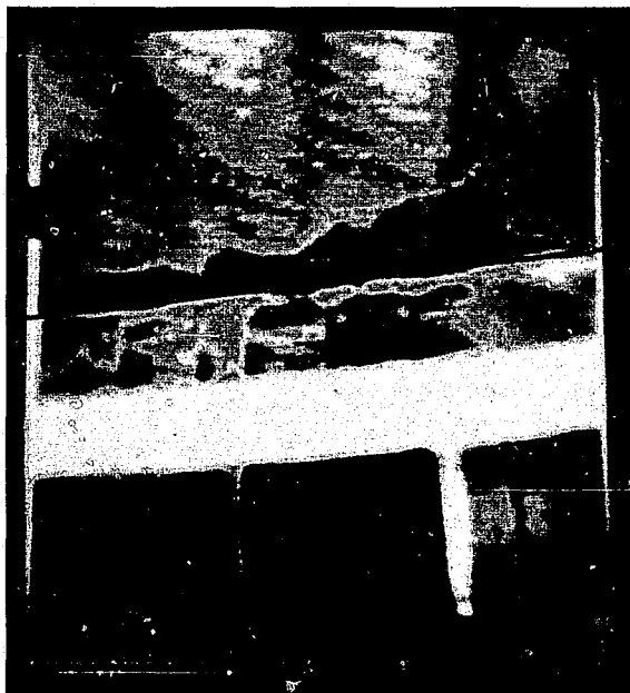
FIGURE B-5. Interior view of ceiling-wall interface above the bay window in living room. (b) Thermogram before retrofit.
