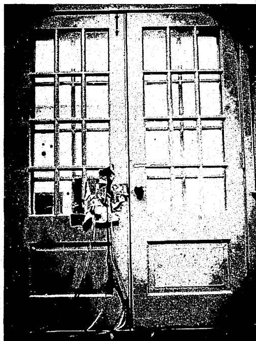
FIGURE B-4. Interior surface of dining room door. (a) Conventional photograph.
