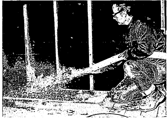
FIGURE A-2. Loose-fill cellulose being blown on top of the existing ceiling insulation.
