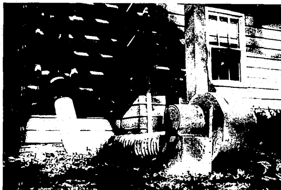
FIGURE C-3. Centrifugal blower connected to the window panel with a flexible hose.
