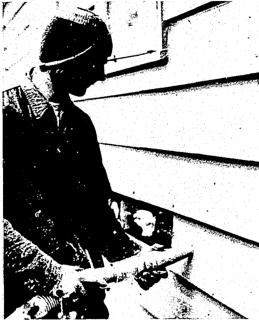
FIGURE A-3. Cellulosic fiber being blown into the walls of the test house.
