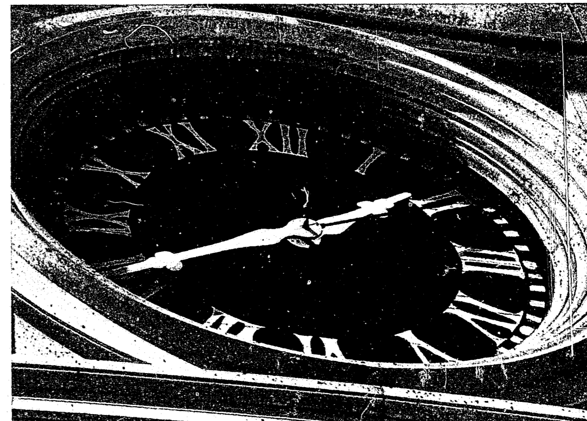
As part of the restoration of Ali'iolani Hale, the clock tower atop the building is being repaired. It was installed in 1874 at the cost of $400, and the clock still has its original works.
