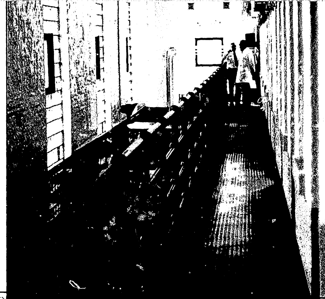
Above: New fire-safe steel flooring was installed in the Restricted Housing Unit at SCI-Pittsburgh, replacing old wooden floor at a cost of $13,675. Inmate and staff labor made for a total savings of $11,000 to taxpayers.
