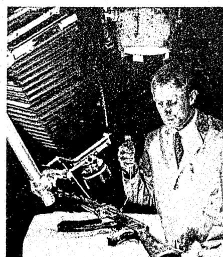
A serial number which had been ground off the weapon is restored and then photographed.
