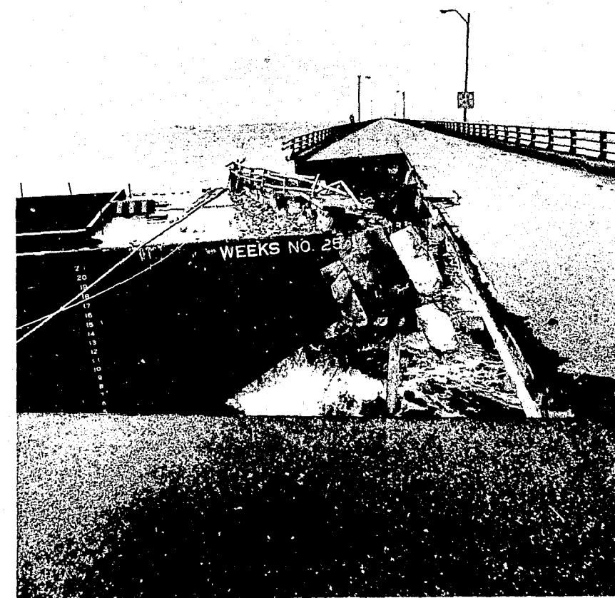
Without warning, a converted powerless barge struck the bridge span, closing the bridge-tunnel to traffic for several days. Photo: Studio III, Norfolk, Va.
