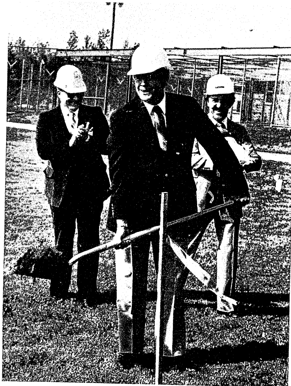
September 21, 1982 — Gov. Richard A. Snelling turns the first shovelful of dirt for the construction of the Vermont Institutional Industries on-site work program building at the Northwest State Correctional Facility in St. Albans.
