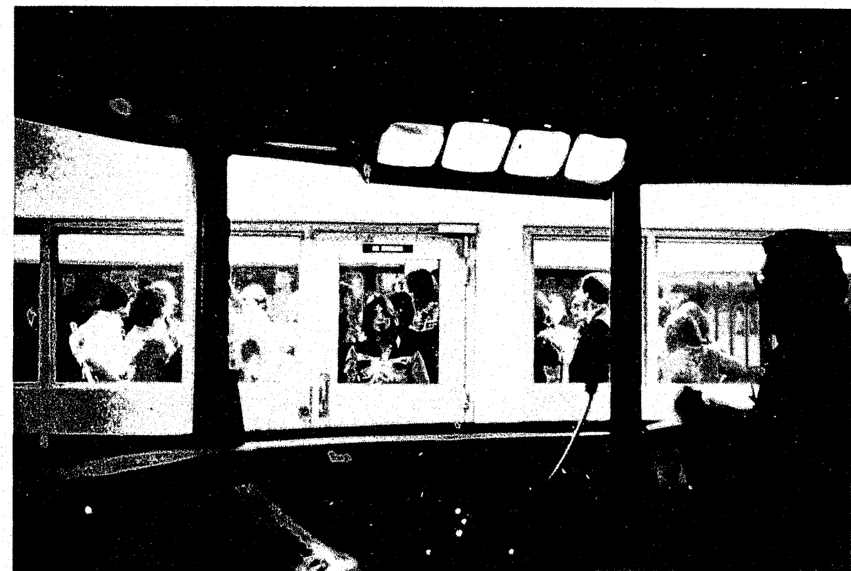
Central control room at the new St. Johnsbury Correctional Center. This is the nerve center of the facility from which the operator can monitor and control all movement of inmates.
