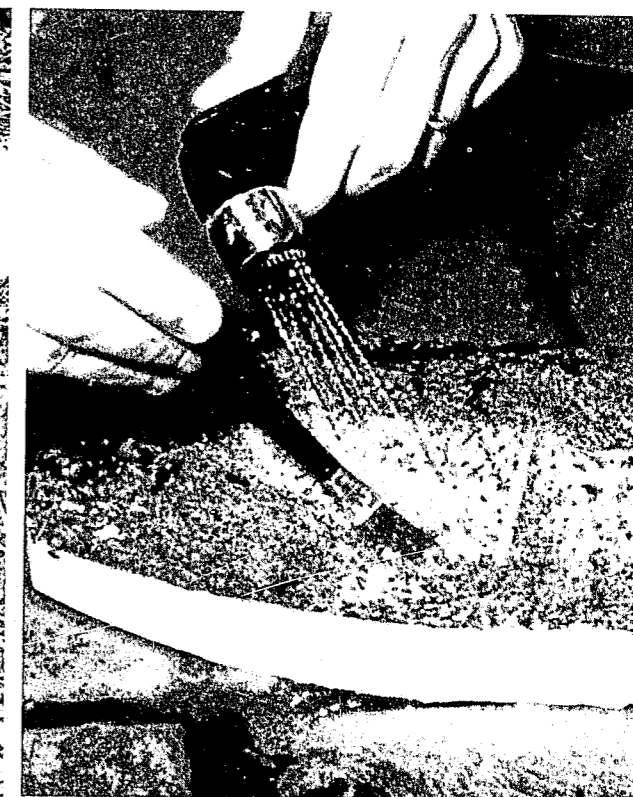
Removing dirt and debris with water and brush.
