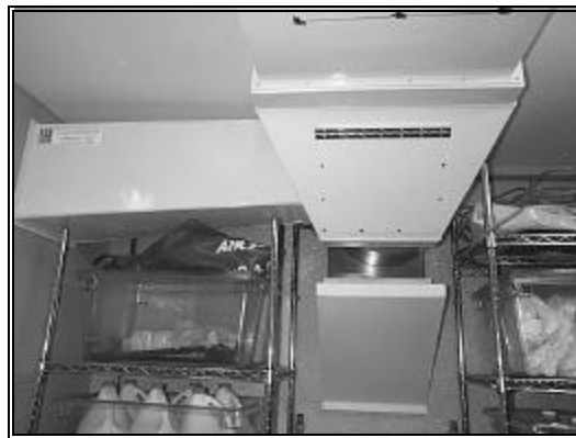
Figure 5. Section 4, storage area
