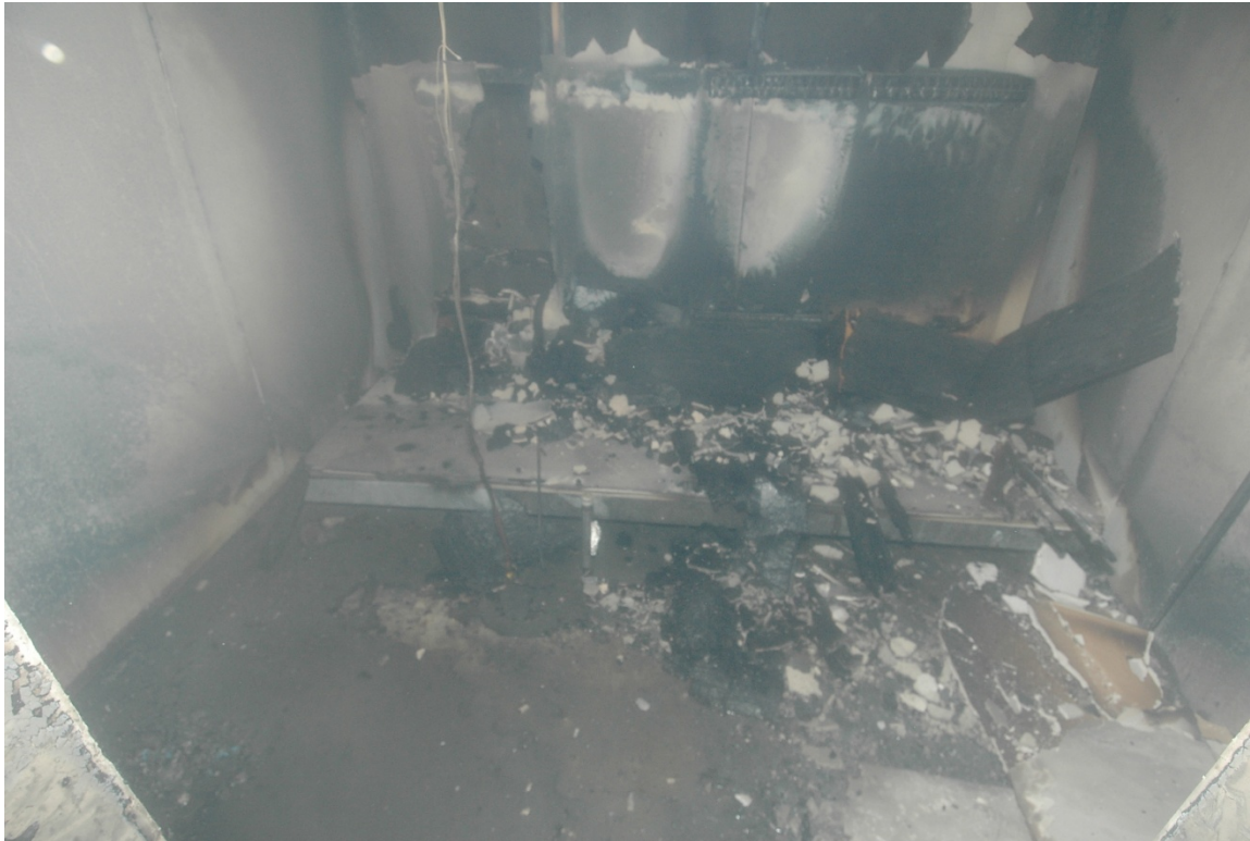
Figure 8-10. Fire pattern from test CL3 (open door)
