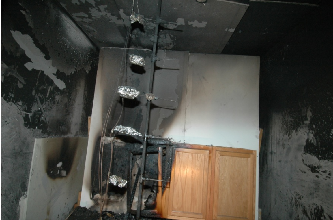
Figure 8-8. Fire pattern from test CL1 (no ventilation)
