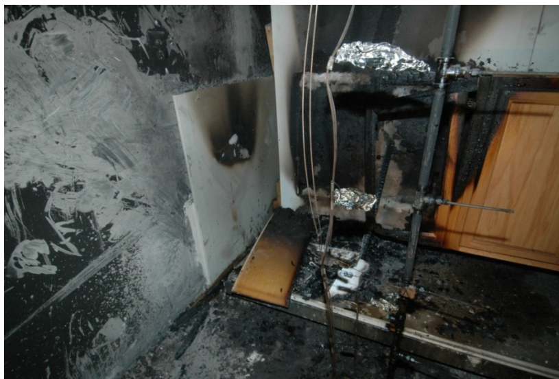
Figure 5-33. Test CL1 damage – low cabinets with no ventilation.
