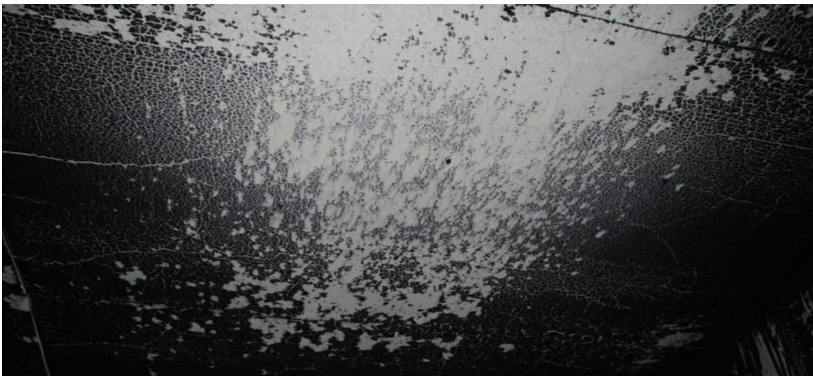
Figure 96. Pattern identified on the ceiling of the enclosure after Test 6-5.
