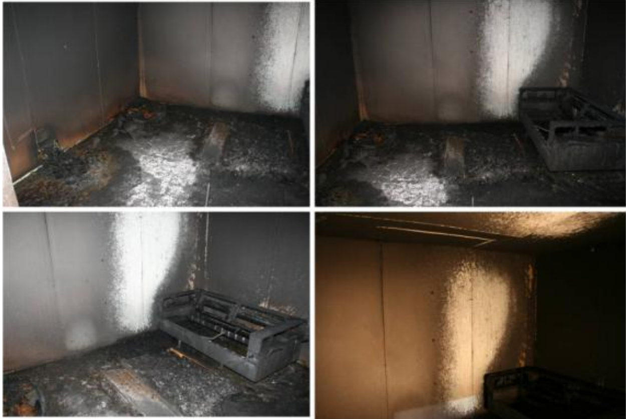
Figure 62. Enclosure conditions after Test 6-1.
