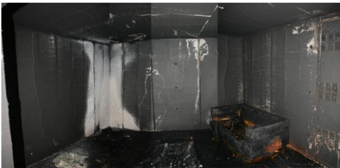
Figure 111. Composite photograph of enclosure conditions after Test 6-8.
