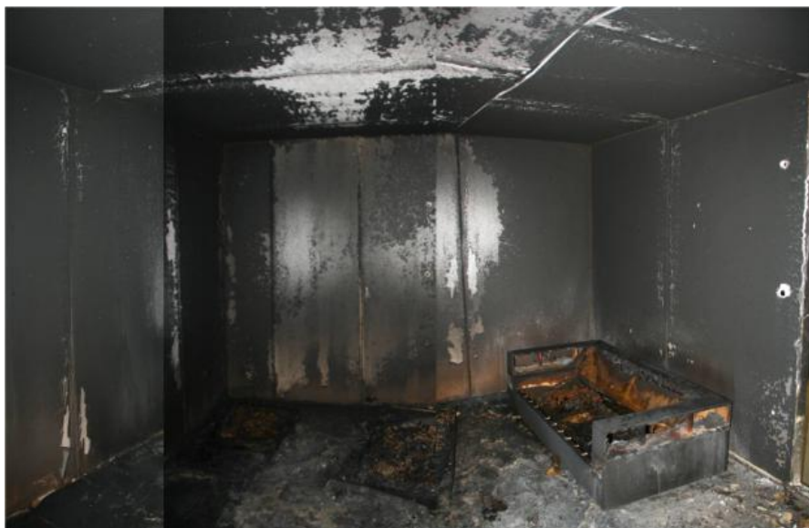
Figure 31. Condition of enclosure ceiling after Test 6-7.
