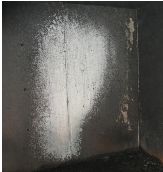
Figure 64. Close up photograph of wall pattern identified in Test 6-1.
