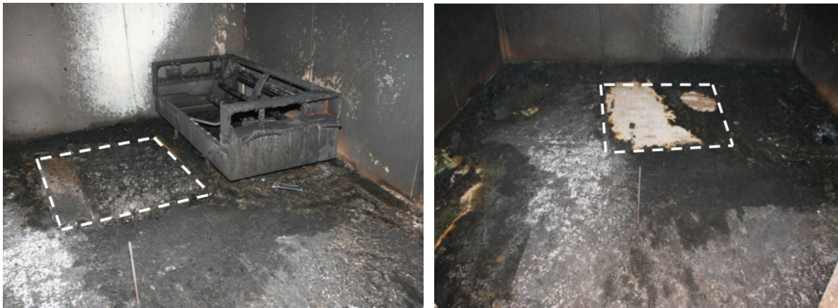
Figure 130. Condition of wooden table and flooring after Test 6-1 prior to overhaul (left) and after overhaul (right).
