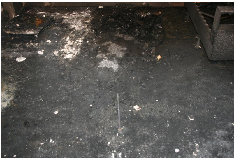
Figure 84. Condition of carpet flooring after Test 6-3.
