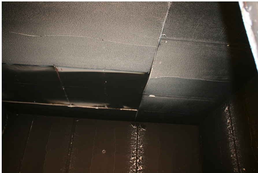
Figure 81. Condition of ceiling after Test 6-3.
