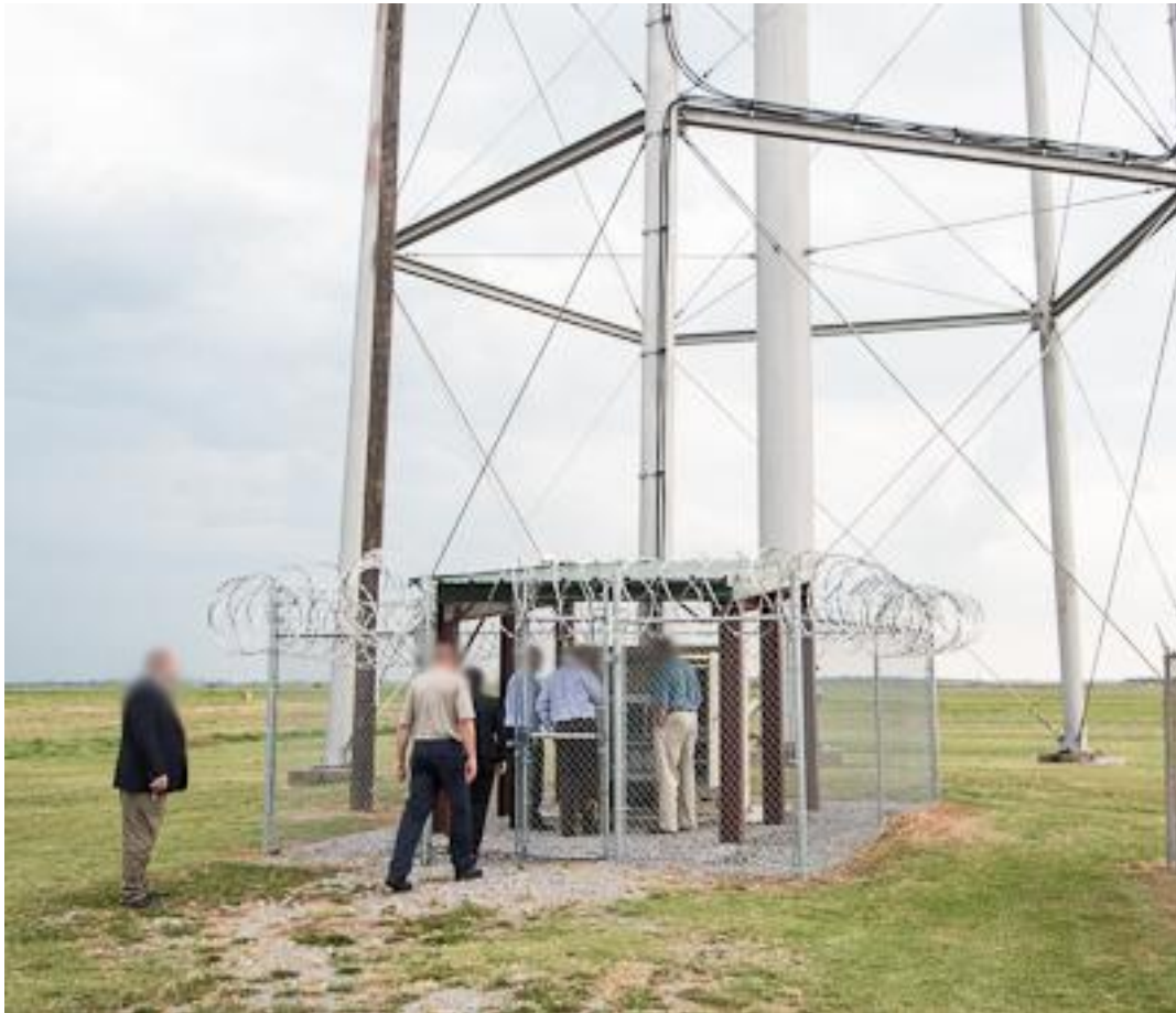
Figure 16. The MDOC Water Tower Equipment shelter
